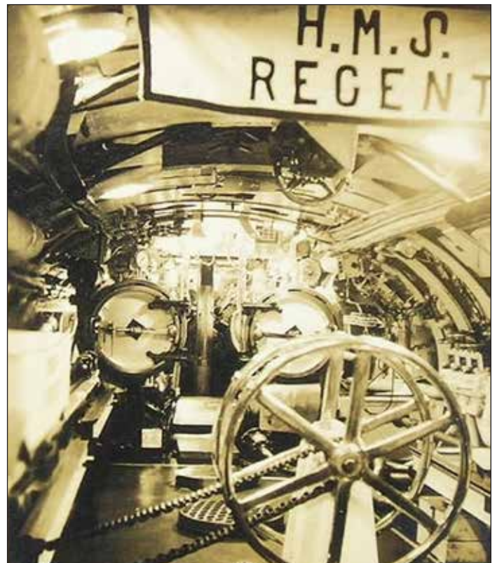
The interior of HMS Regent, looking toward the torpedo tubes.
